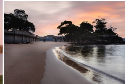
Rocky Point Island Bridge Credit - Set Subject Cushla Monk
