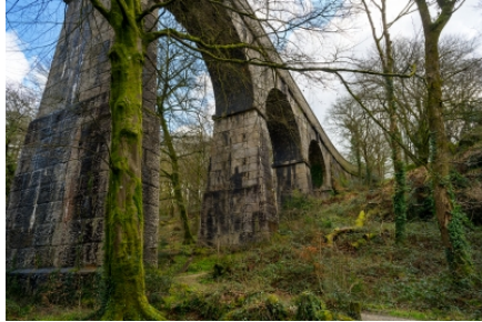
Treffry Viaduct Cornwall
